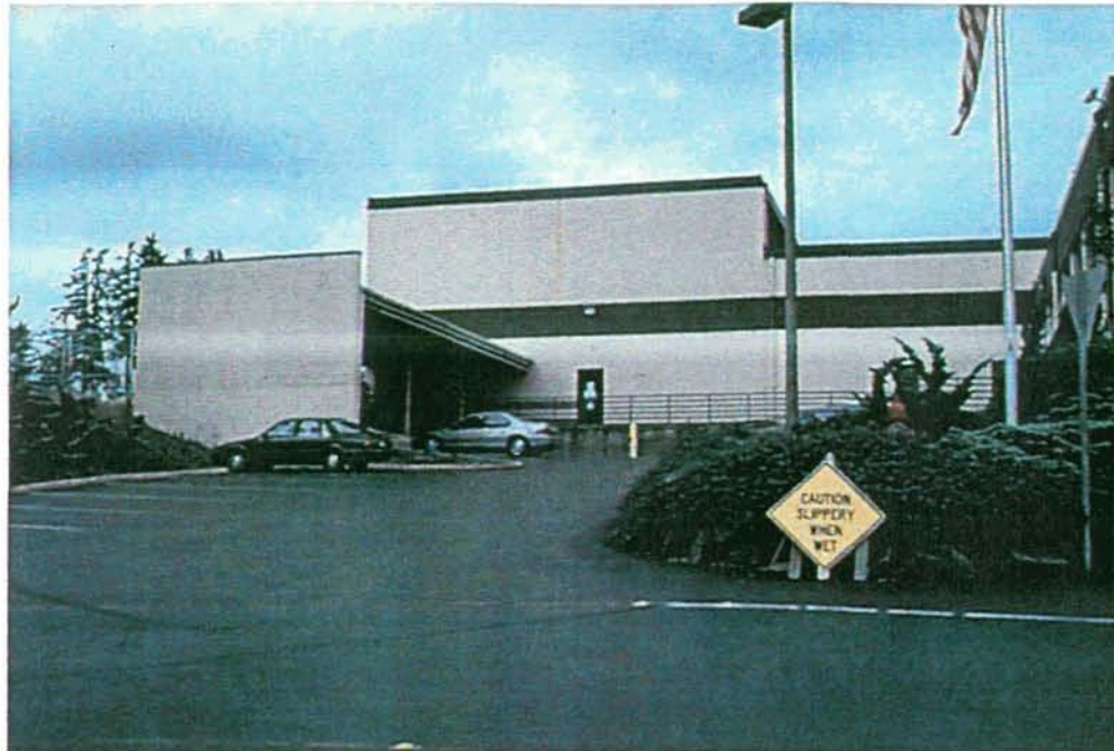
PHOTO #1 - SOUTHEAST SIDE VIEW OF FACILITY
