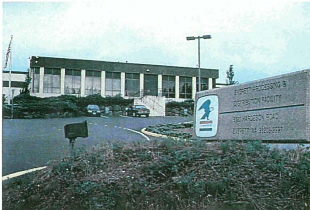
PHOTO #2 - EAST SIDE VIEW OF FACILITY WITH TRANSITE PANELS ABOVE WINDOWS
