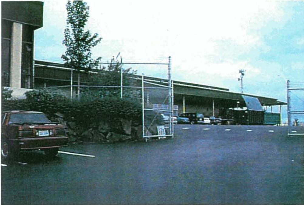
PHOTO #3 - NORTHEAST SIDE VIEW OF FACILITY
