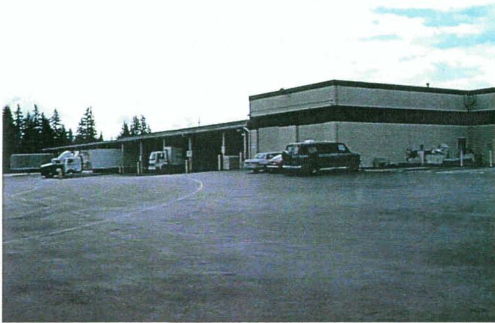
PHOTO #4 - NORTH SIDE VIEW OF FACILITY
