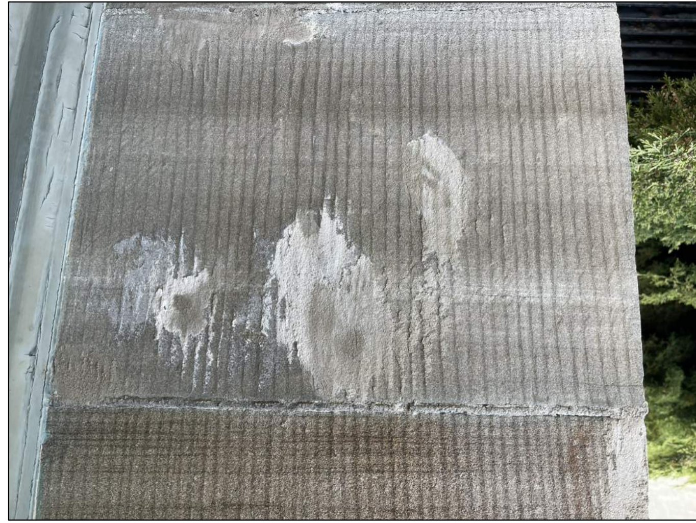
1 PREVIOUS PATCH AT JAMB SCALE: NTS
