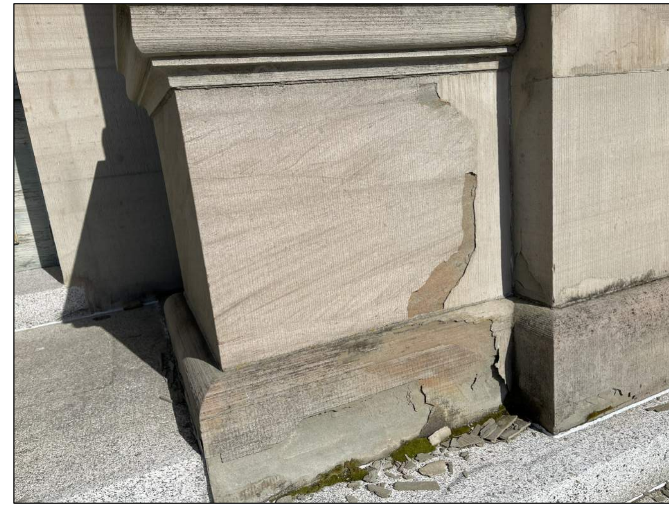
3 SPALLING AT COLUMN BASE SCALE: NTS
