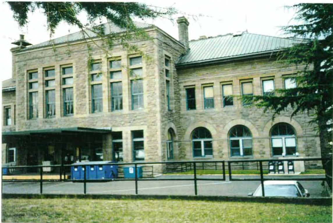
Metal Roof Vapor Barrier and Rolled Roof Not Sampled Assumed ACBM
