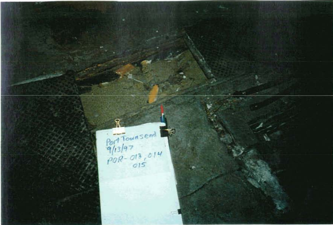
Trench Insulation and Debris Sample Number: 013, 014, 015 Homogeneous Material Photograph
