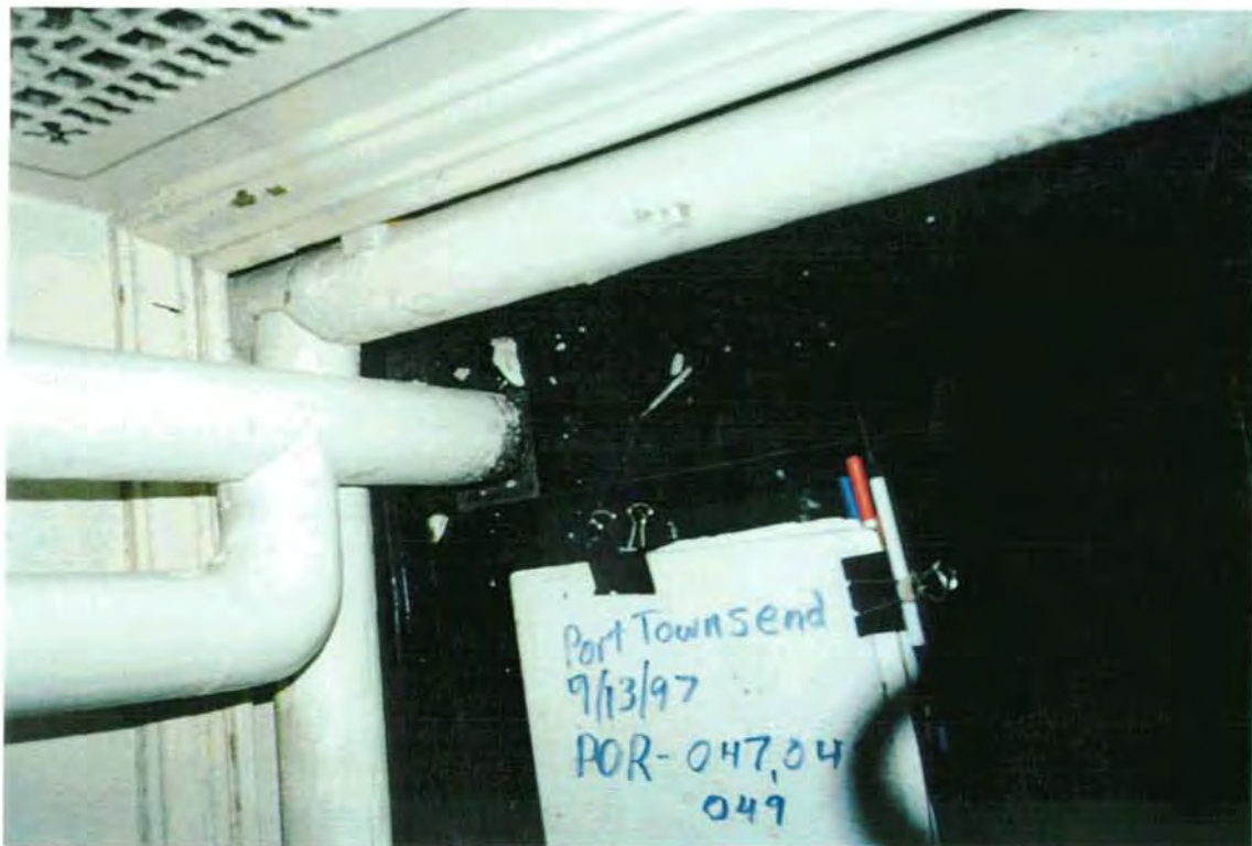
12"x12" Brown Floor Tile and Mastic under 12"x12" Black Floor Tile Sample Number: 047,048,049 Homogeneous Material Photograph
