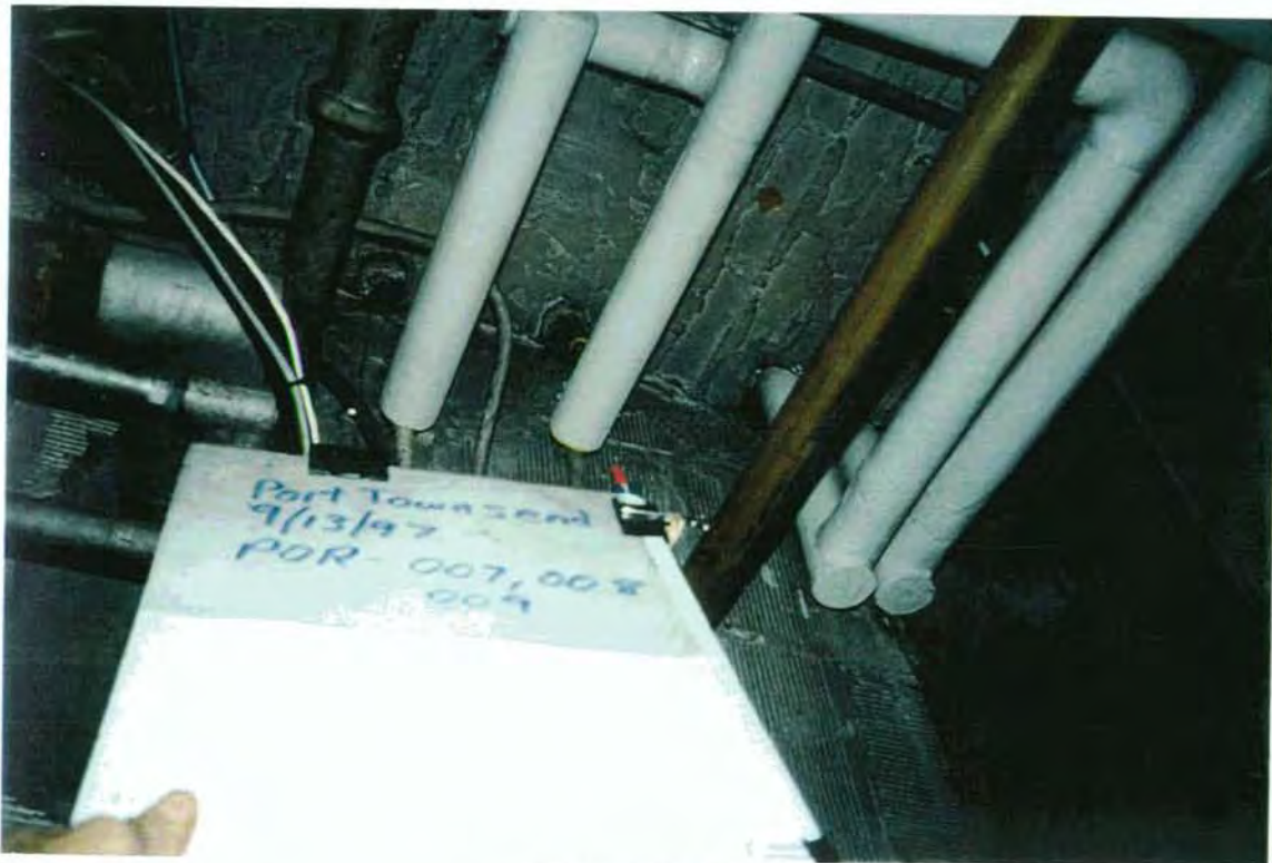
Pipe Insulation Ends Sample Numbers: 007,008,009,116 Homogeneous Material Photograph
