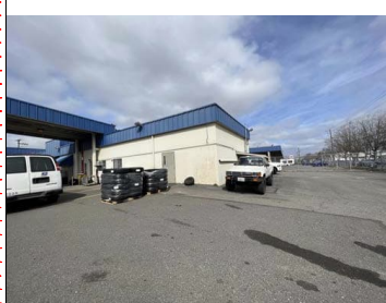
5 PHOTOGRAPH - EXTERIOR OF VMF BUILDING AT SOUTH EAST ELEVATION
