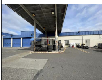
4 PHOTOGRAPH - EXTERIOR OF VMF BUILDING AT CANOPY
