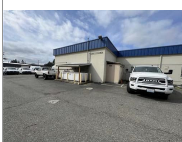
7 PHOTOGRAPH - EXTERIOR OF VMF BUILDING AT EAST ELEVATION
