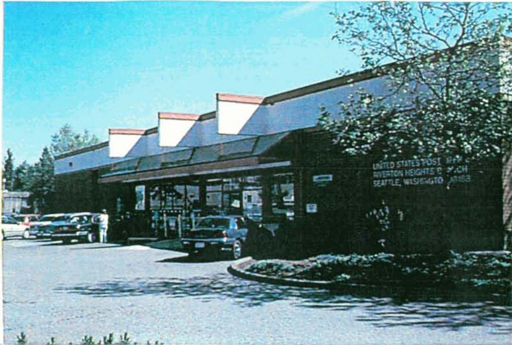
PHOTO #1 - FRONT OF FACILITY
