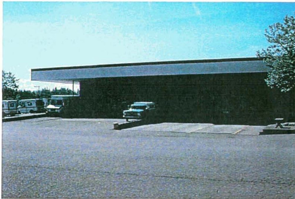
PHOTO #2 - REAR OF FACILITY
