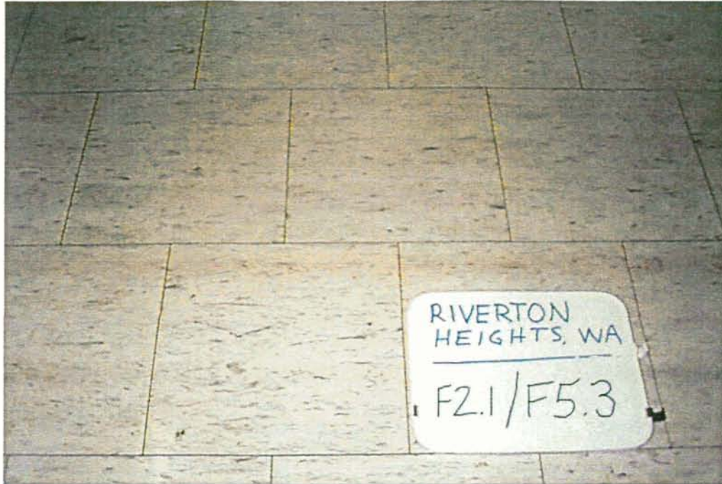
PHOTO #3 - 12"x12" CREAM FLOOR TILE (F2.1) AND MASTIC (F5.3)
