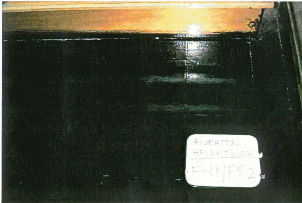
PHOTO #4 - 12"x24" BLACK FLOOR PLANK (F4.1) AND MASTIC (F5.2)
