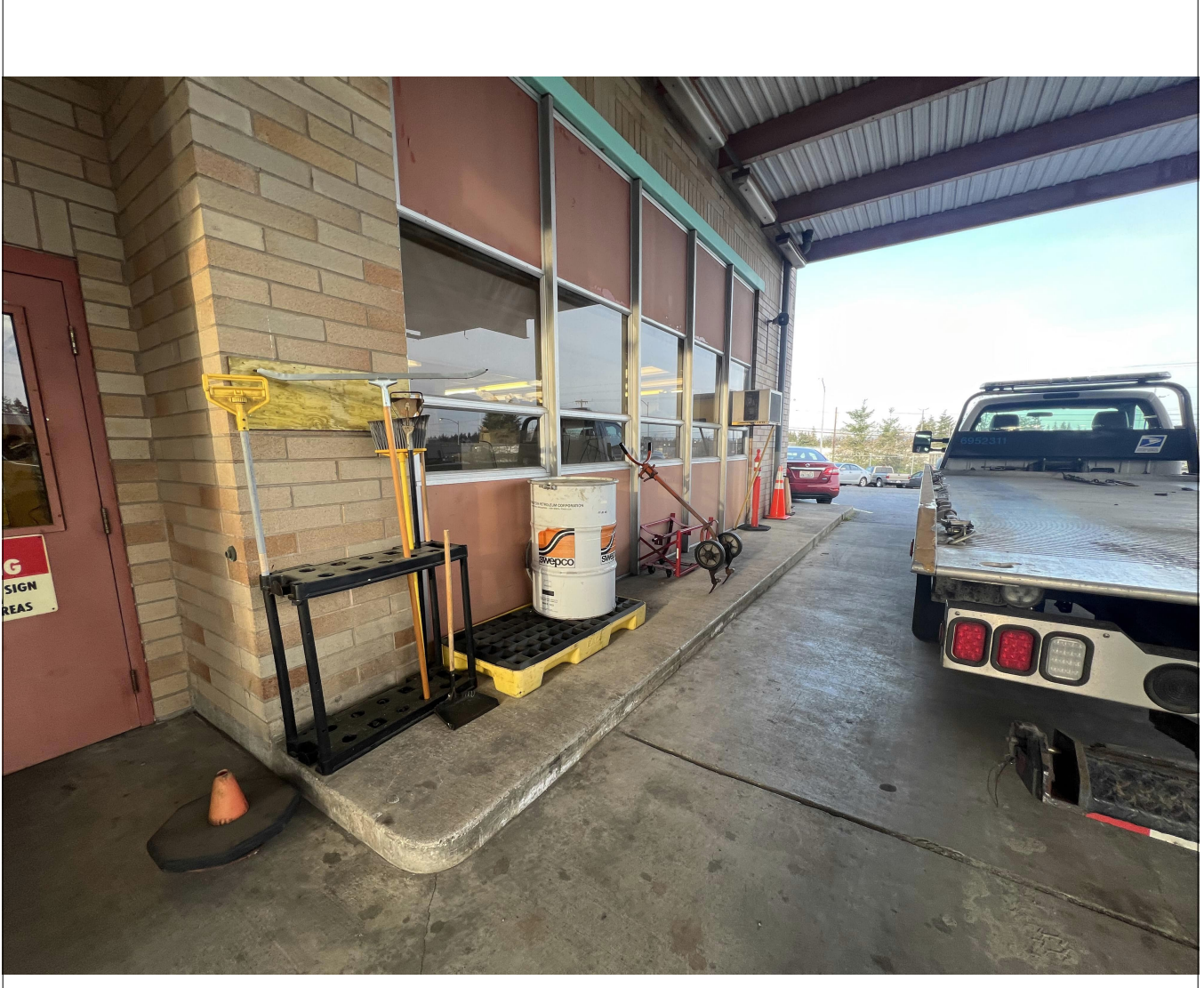
Detail: Fac. | Ch. | Sect. | Para. | Detail CAD File: Scale: USPS SDL Issued: Last Revised:
