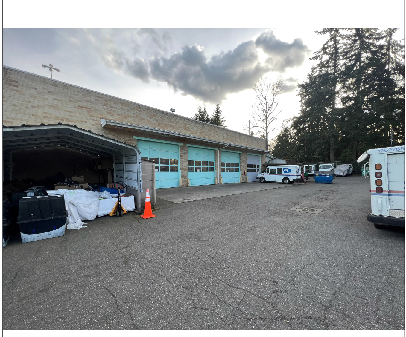
Detail: Fac. | Ch. | Sect. | Para. | Detail CAD File: Scale: USPS SDL Issued: Last Revised:
