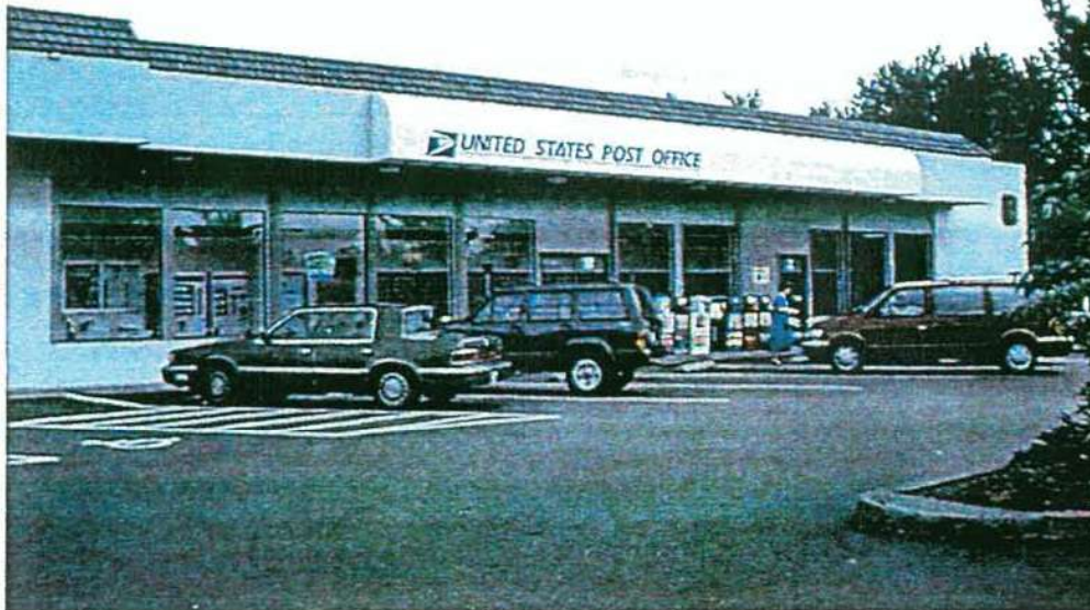
PHOTO #1 - FRONT OF FACILITY
