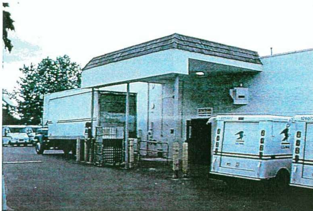
PHOTO #2 - REAR OF FACILITY
