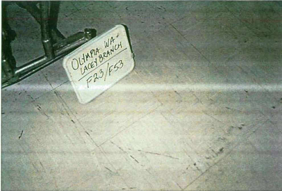
PHOTO #5 - MASTIC UNDER 12"x12"
