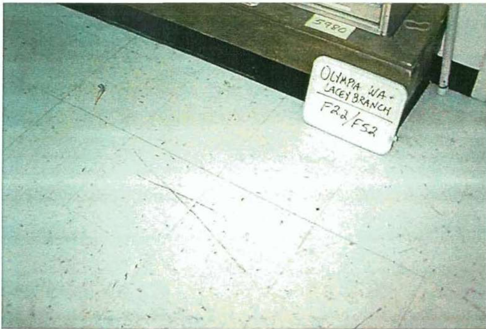
PHOTO #4 - 12"x12" BEIGE WITH BROWN SPOTS FLOOR TILE (F2.2) AND MASTIC (F5.2)
