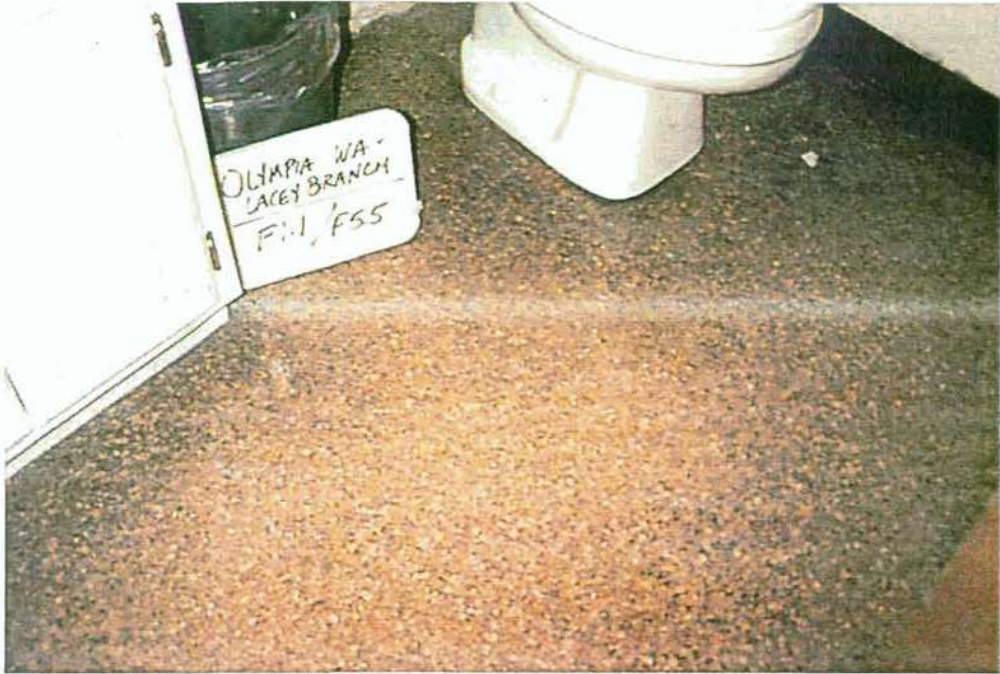
PHOTO #3 - GOLD SHEET VINYL (F1.1) AND MASTIC (F5.5)
