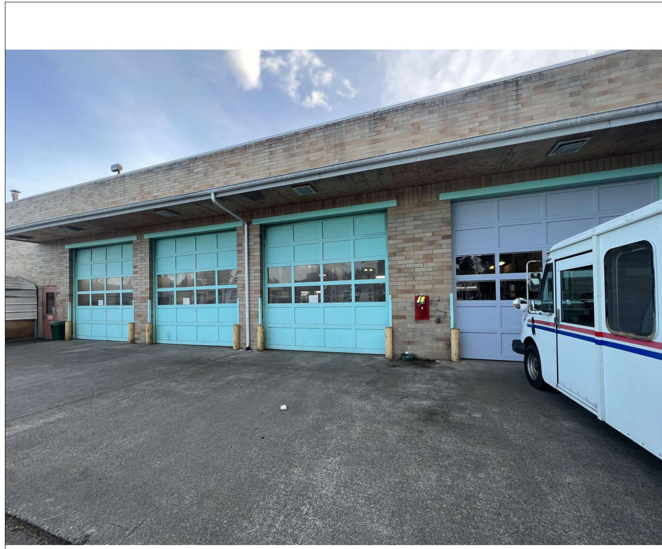
3 EXTERIOR OF VMF AT NORTH FACADE
