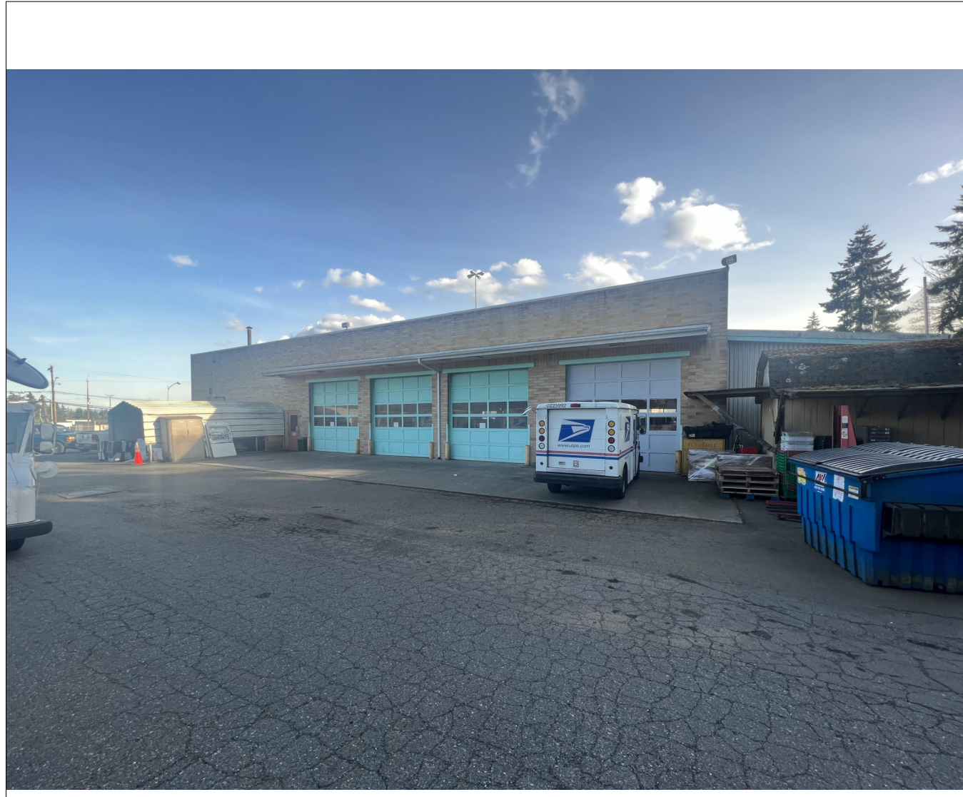
7 EXTERIOR OF VMF AT NORTH FACADE
