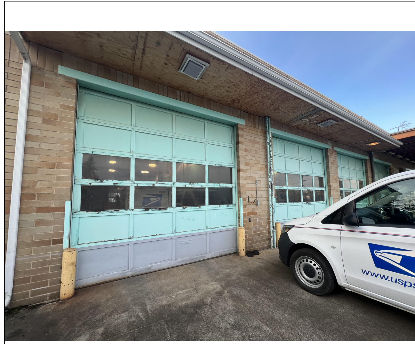
4 EXTERIOR OF VMF AT SOUTH FACADE
