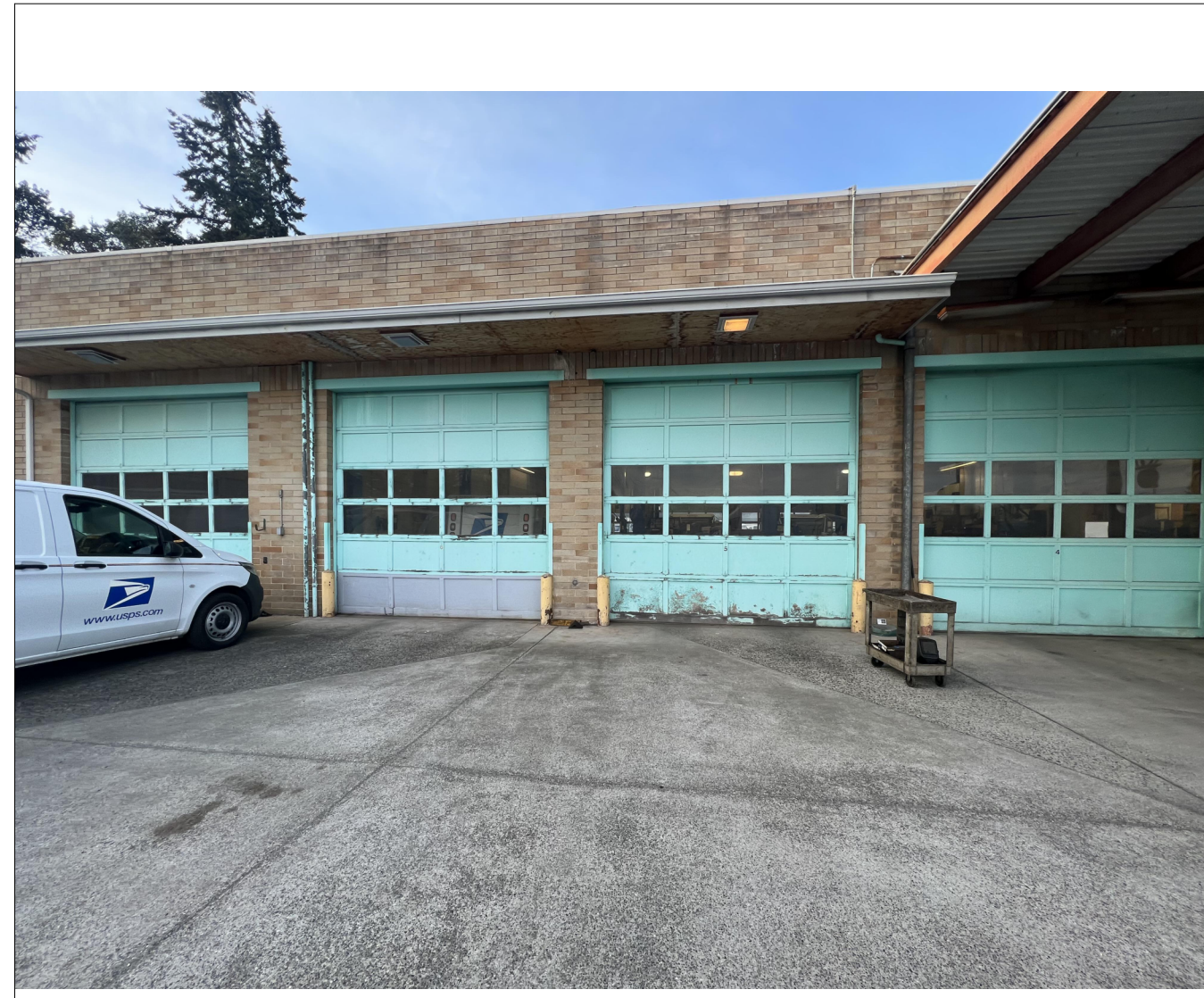
5 EXTERIOR OF VMF AT SOUTH FACADE
