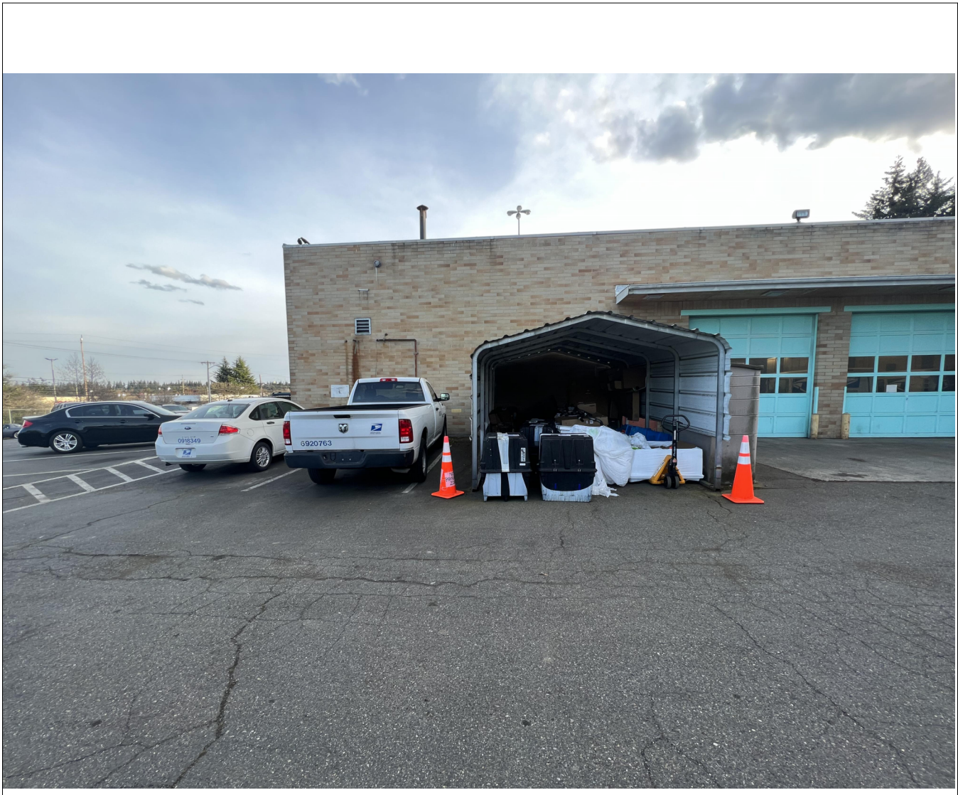
1 EXTERIOR OF VMF AT NORTH FACADE
