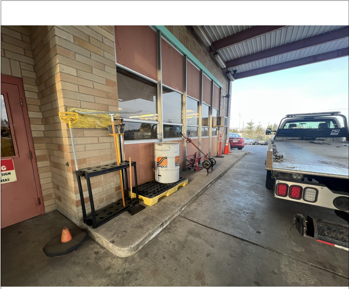
6 EXTERIOR OF VMF AT SOUTH FACADE
