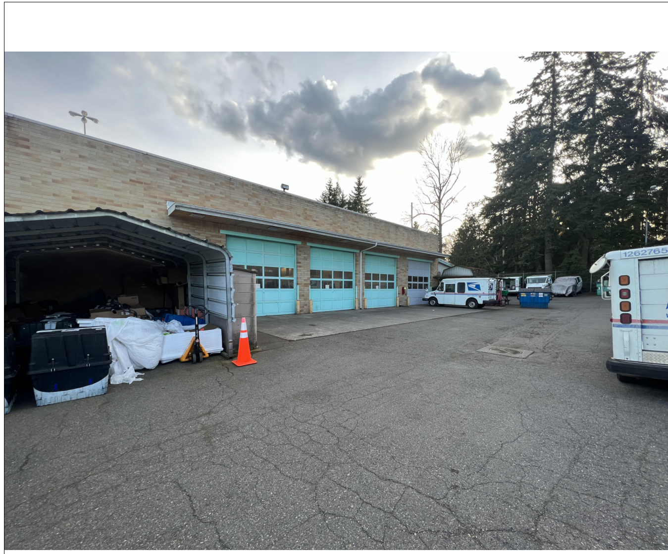
2 EXTERIOR OF VMF AT NORTH FACADE
