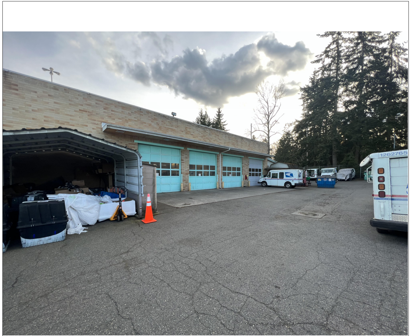
2 EXTERIOR OF VMF AT NORTH FACADE
