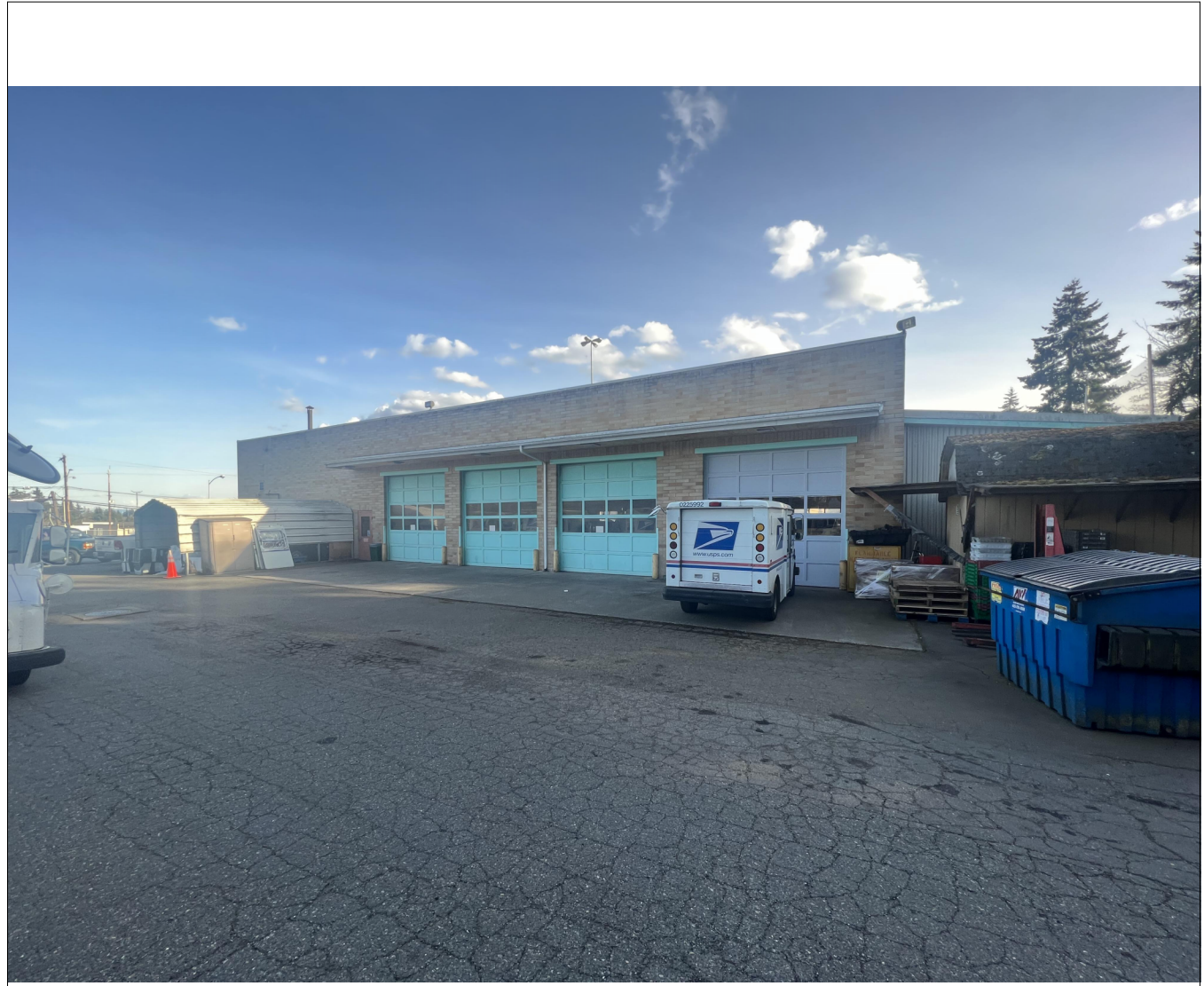
7 EXTERIOR OF VMF AT NORTH FACADE
