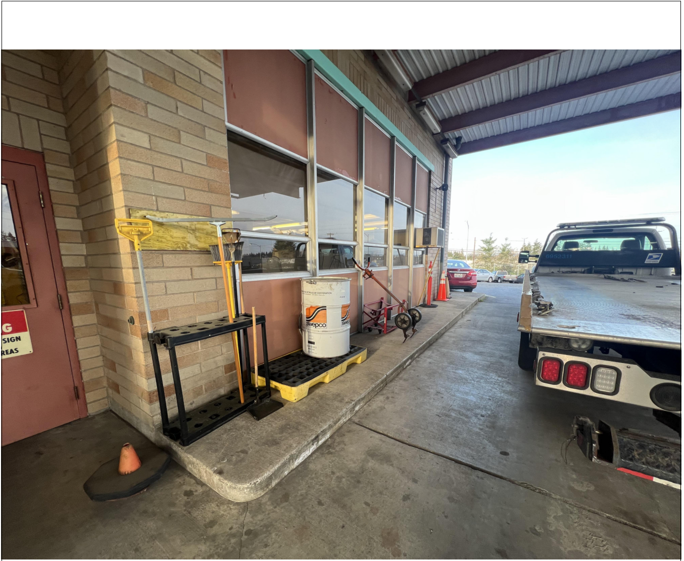
6 EXTERIOR OF VMF AT SOUTH FACADE
