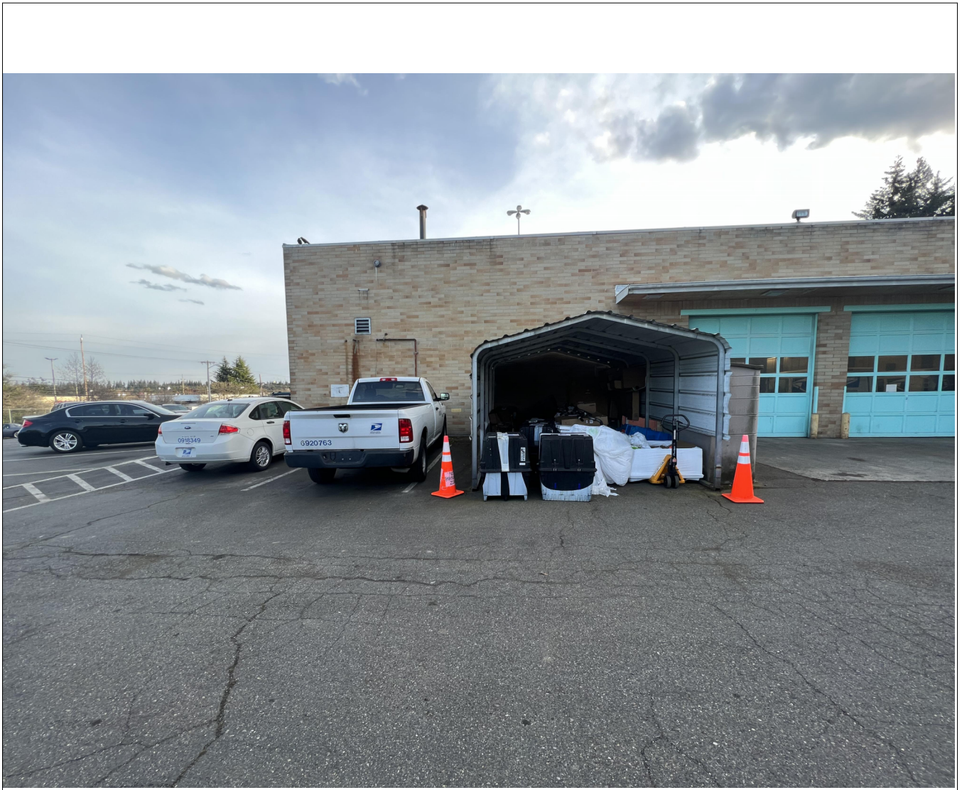
1 EXTERIOR OF VMF AT NORTH FACADE
