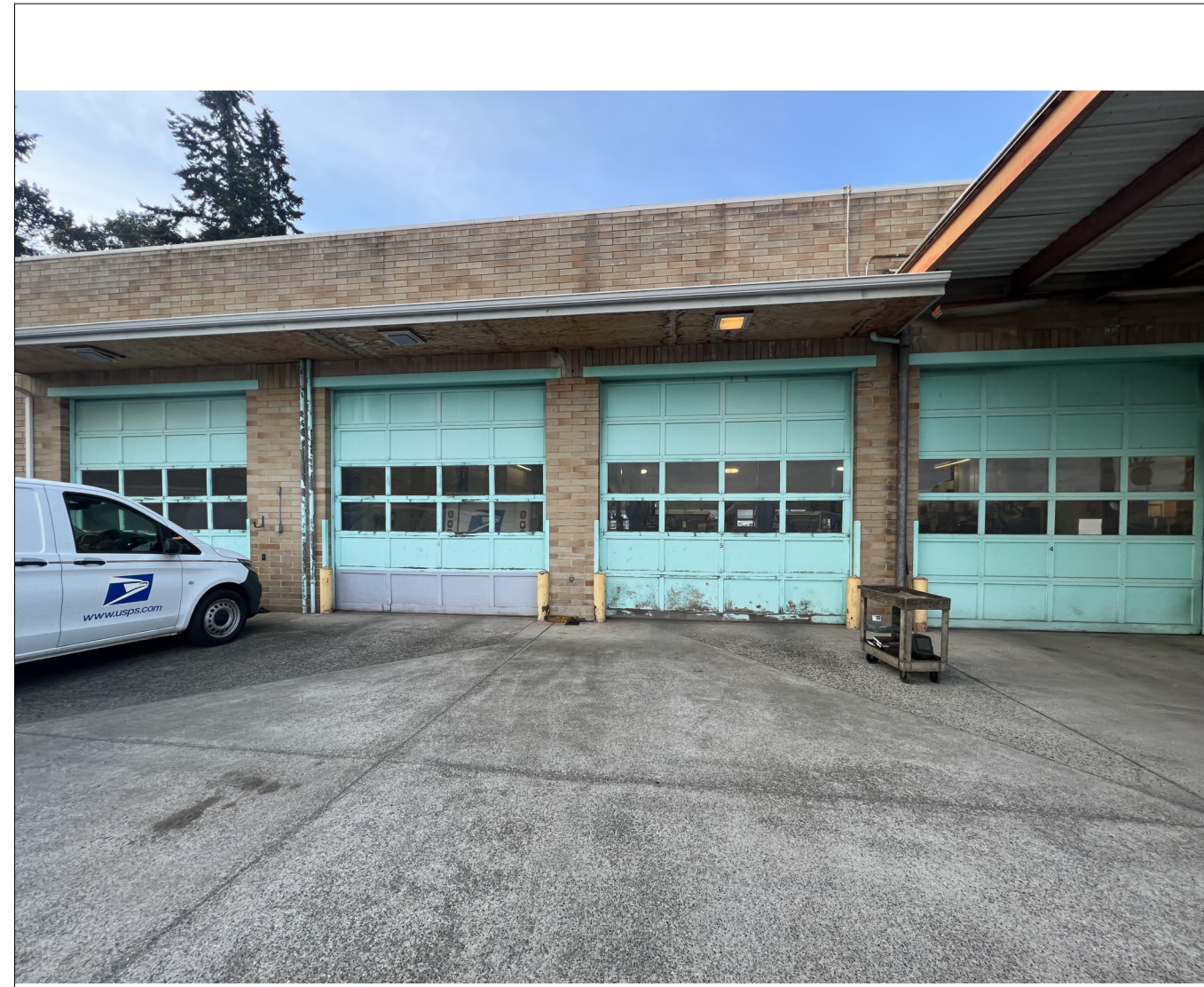
5 EXTERIOR OF VMF AT SOUTH FACADE
