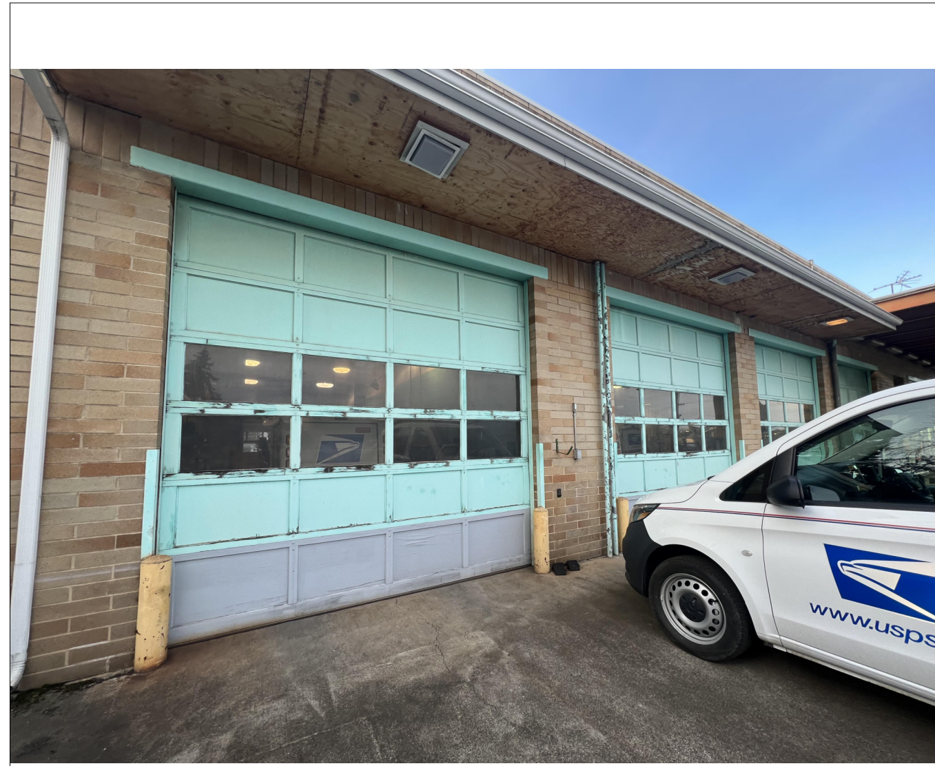
4 EXTERIOR OF VMF AT SOUTH FACADE
