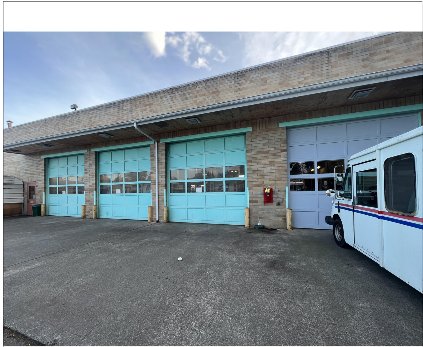
3 EXTERIOR OF VMF AT NORTH FACADE
