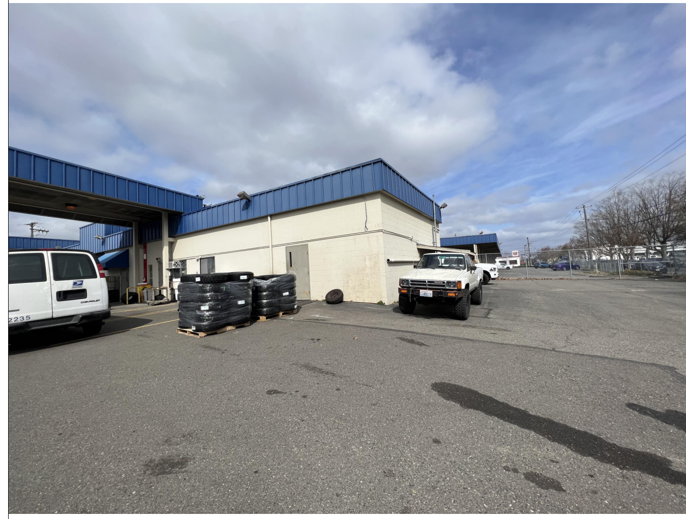
5 PHOTOGRAPH - EXTERIOR OF VMF BUILDING AT SOUTH EAST ELEVATION
