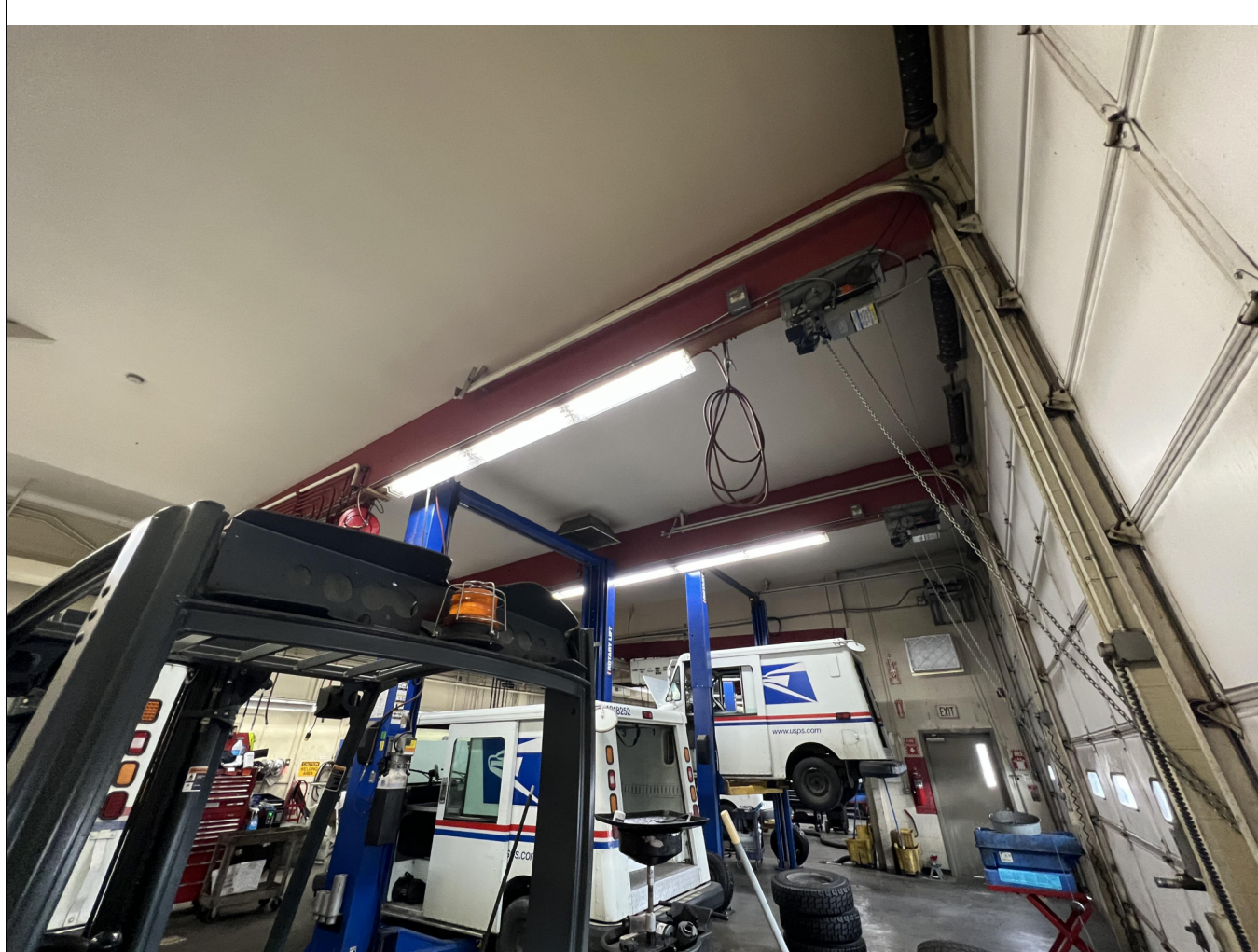
14 PHOTOGRAPH - INTERIOR OF VMF BUILDING AT SERVICE BAY
