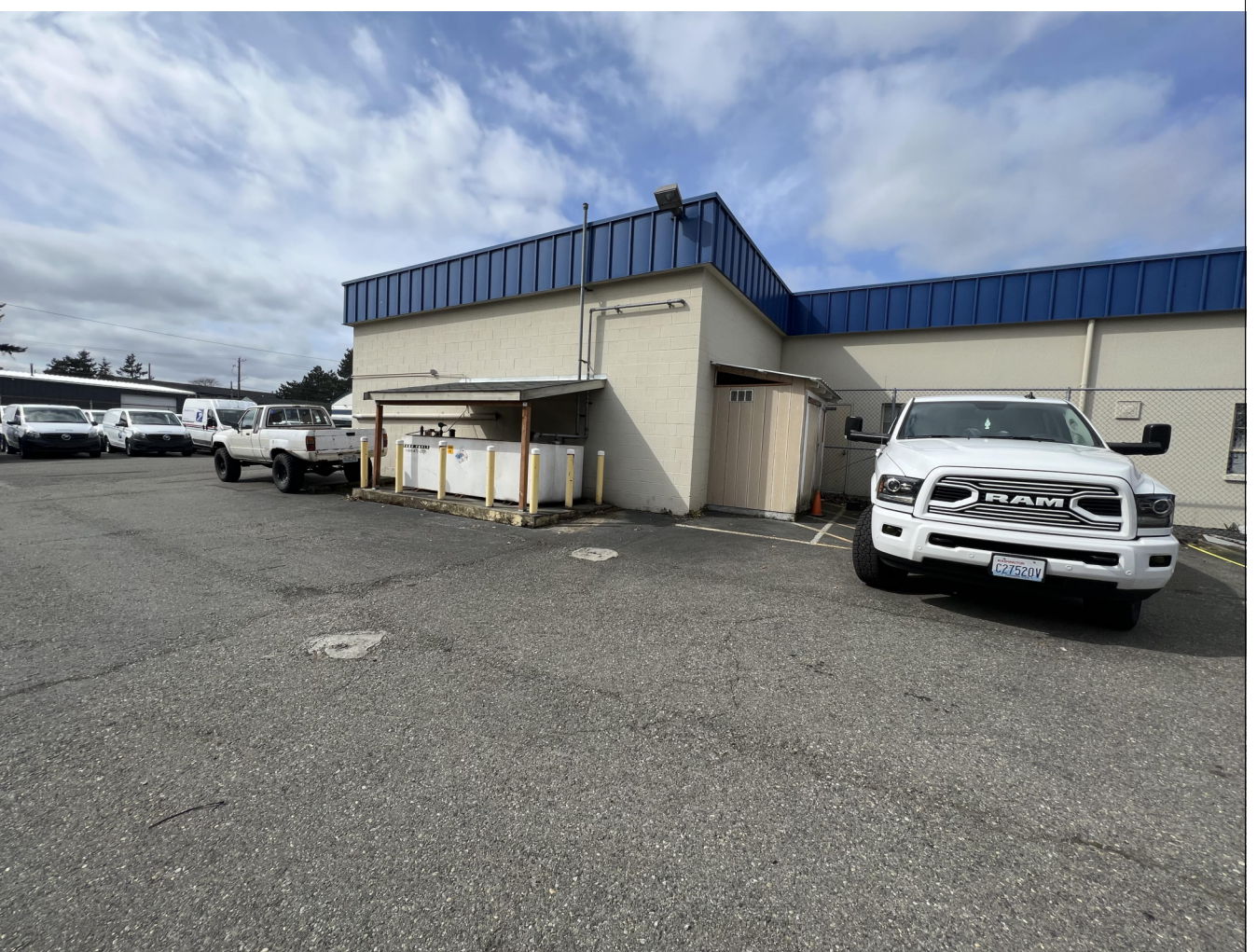
7 PHOTOGRAPH - EXTERIOR OF VMF BUILDING AT EAST ELEVATION
