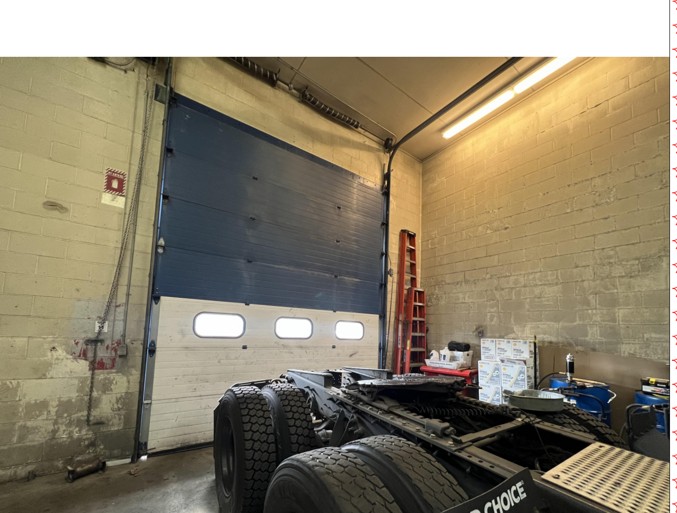
16 PHOTOGRAPH - INTERIOR OF VMF BUILDING AT WASH BAY
