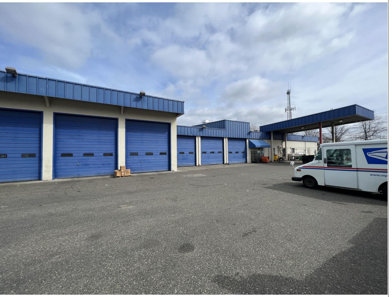
2 PHOTOGRAPH - EXTERIOR OF VMF BUILDING AT SOUTH ELEVATION
