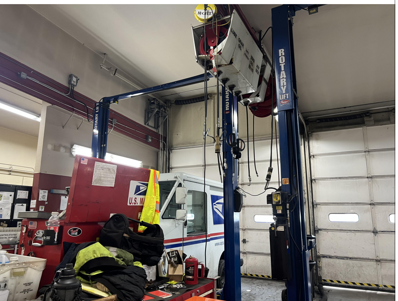
8 PHOTOGRAPH - INTERIOR OF VMF BUILDING AT SERVICE BAY
