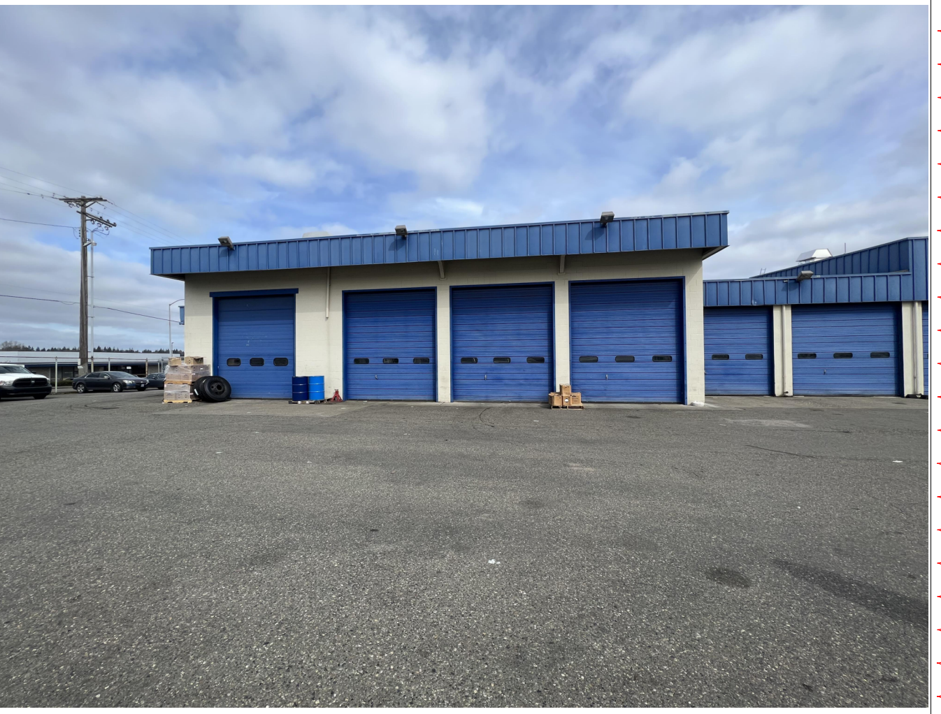
1 PHOTOGRAPH - EXTERIOR OF VMF BUILDING AT SOUTH ELEVATION
