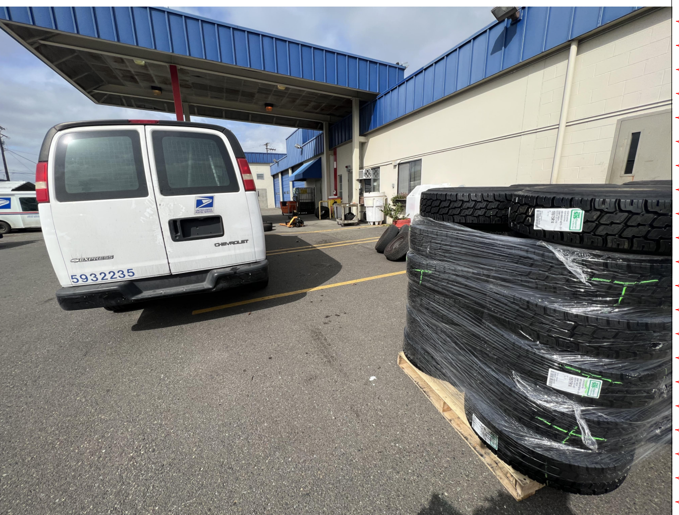
6 PHOTOGRAPH - EXTERIOR OF VMF BUILDING AT SOUTH ELEVATION
