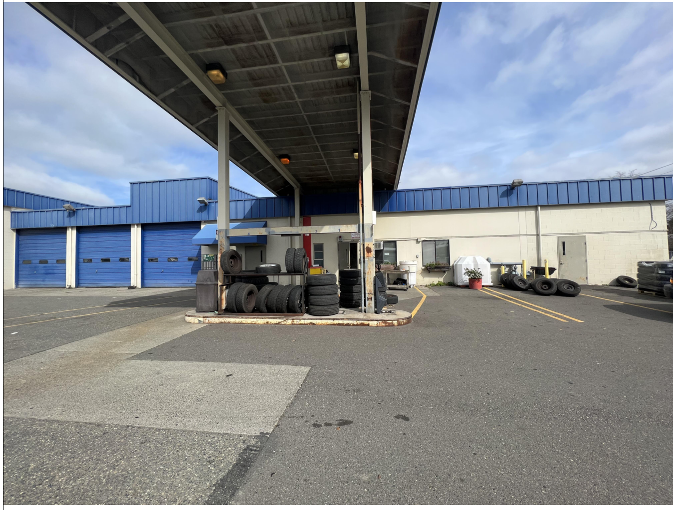
4 PHOTOGRAPH - EXTERIOR OF VMF BUILDING AT CANOPY
