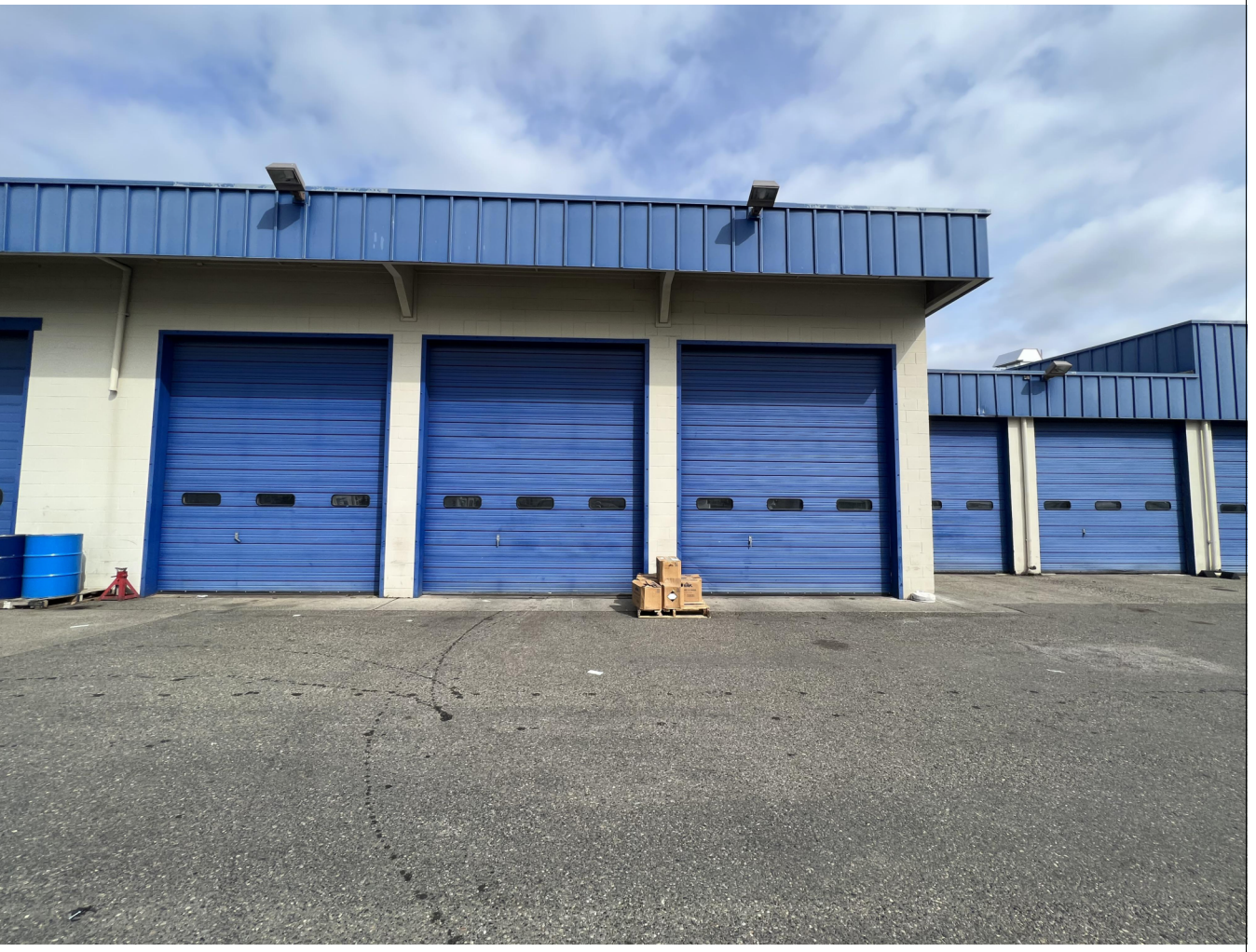
3 PHOTOGRAPH - EXTERIOR OF VMF BUILDING AT SOUTH ELEVATION
